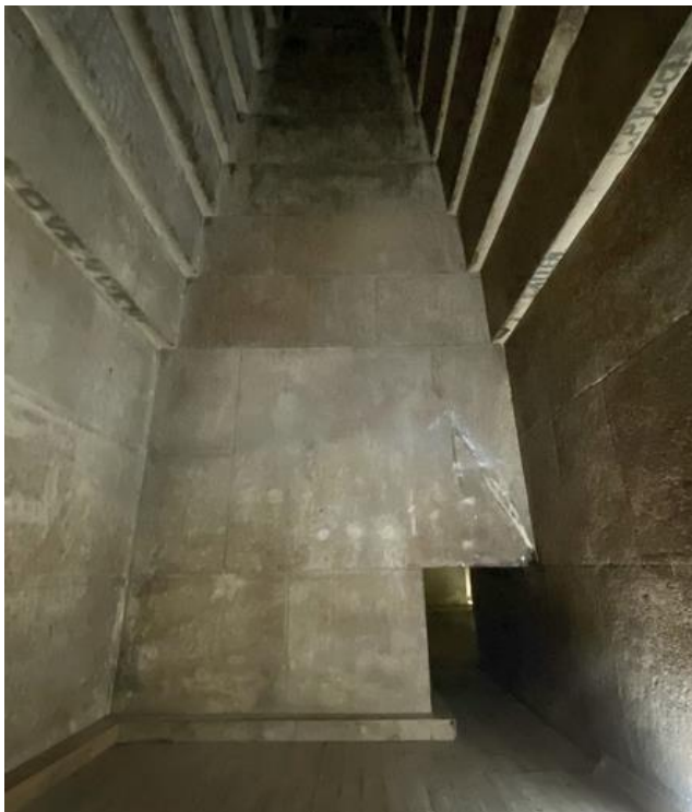
Interior structures of the Red Pyramid (left) and the Bent Pyramid (right) showing the stepped ceiling
